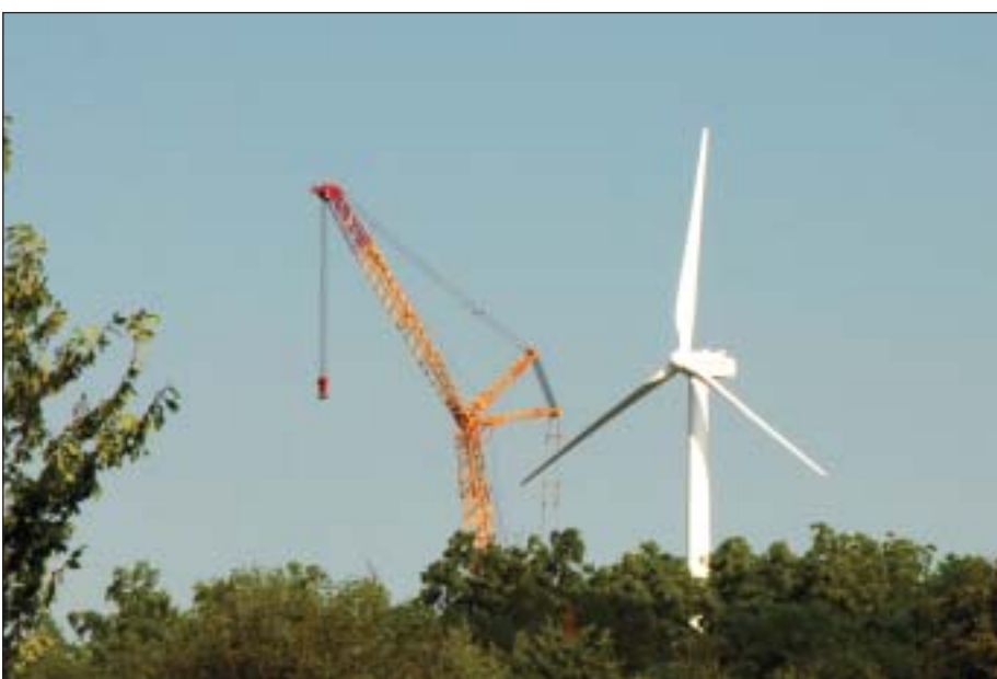
One of many new Wind Trubines along the Rock Port Bluff.
