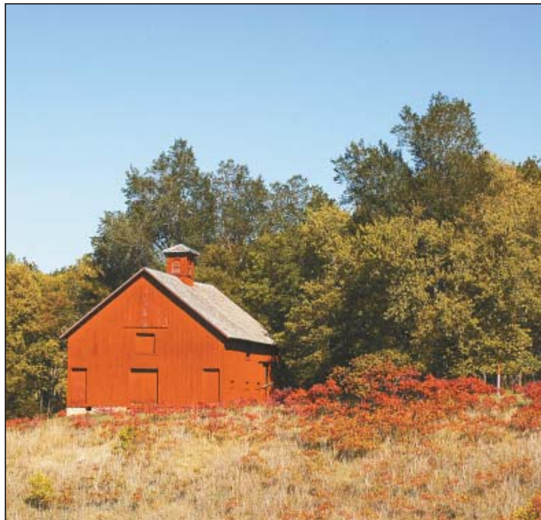
Soley Barn west of Brownville; a different view
