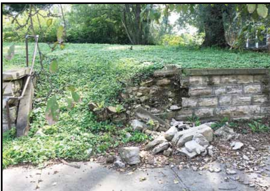
“...some mansions crumble and fall...”
