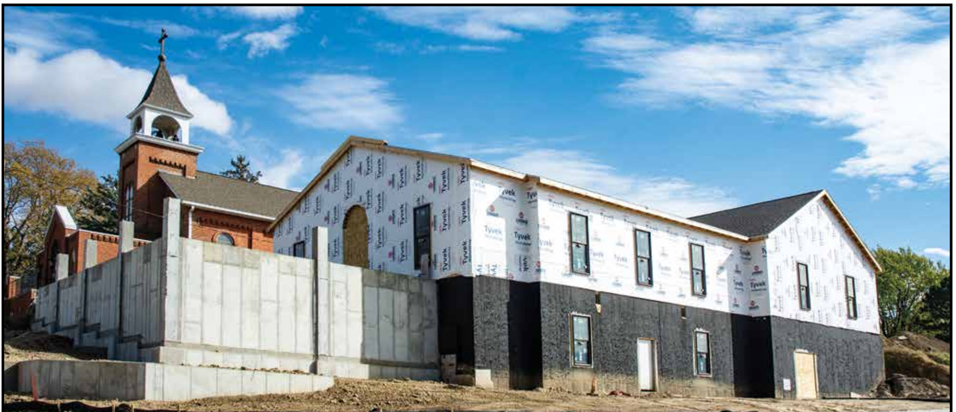
St. Benedict's Community Center is nearing completion.
