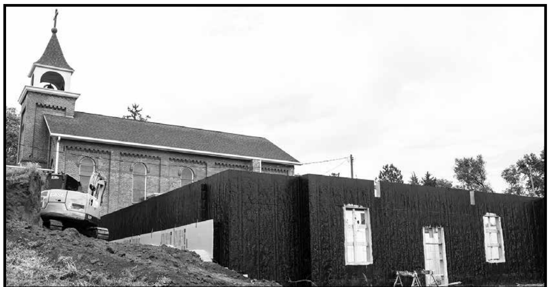
St. Benedict's Community Center Construction, July 2023,
