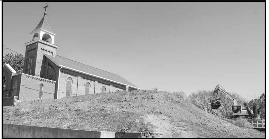
St. Benedict's Community Center Construction, April 2023.
