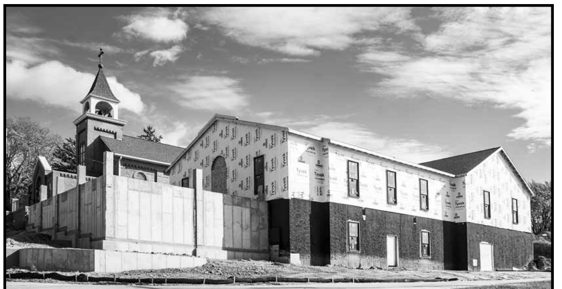
St. Benedict's Community Center Construction, October 24, 2023.
