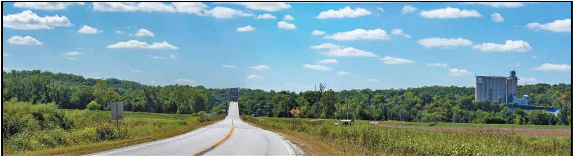
Welcome to Nebraska; Missouri River Bridge ‘gateway’ at Brownville, H-136
