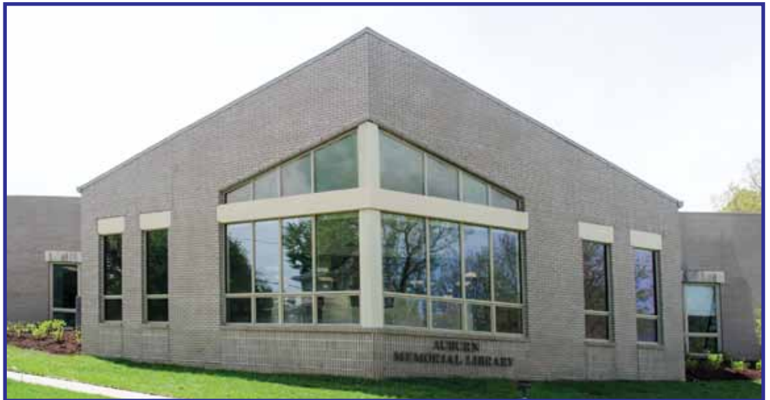
Auburn's library has a new look with the Dorothy Blount Memorial Addition .
