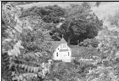
St. Clara's Catholic Church 604 6th Street
