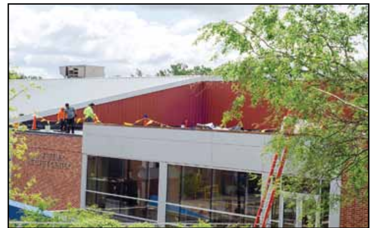
Roof Repairs On The Wheeler Activity Center
