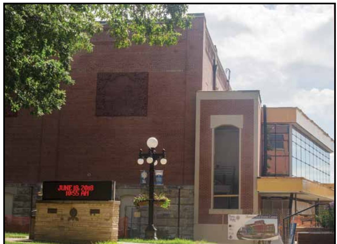
The major construction project on the PSC campus continues to be the Performing Arts Center . Interior work has begun on the project and it is slated to be completed in the Fall of 2018.
