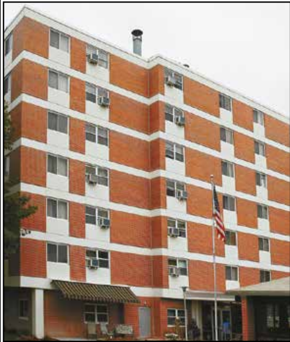
Valley View Apartments (High Rise) • 1017 H Street • Auburn, NE
