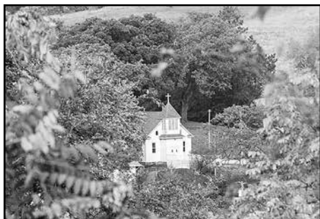
St. Clara’s Catholic Church 604 6th Street
