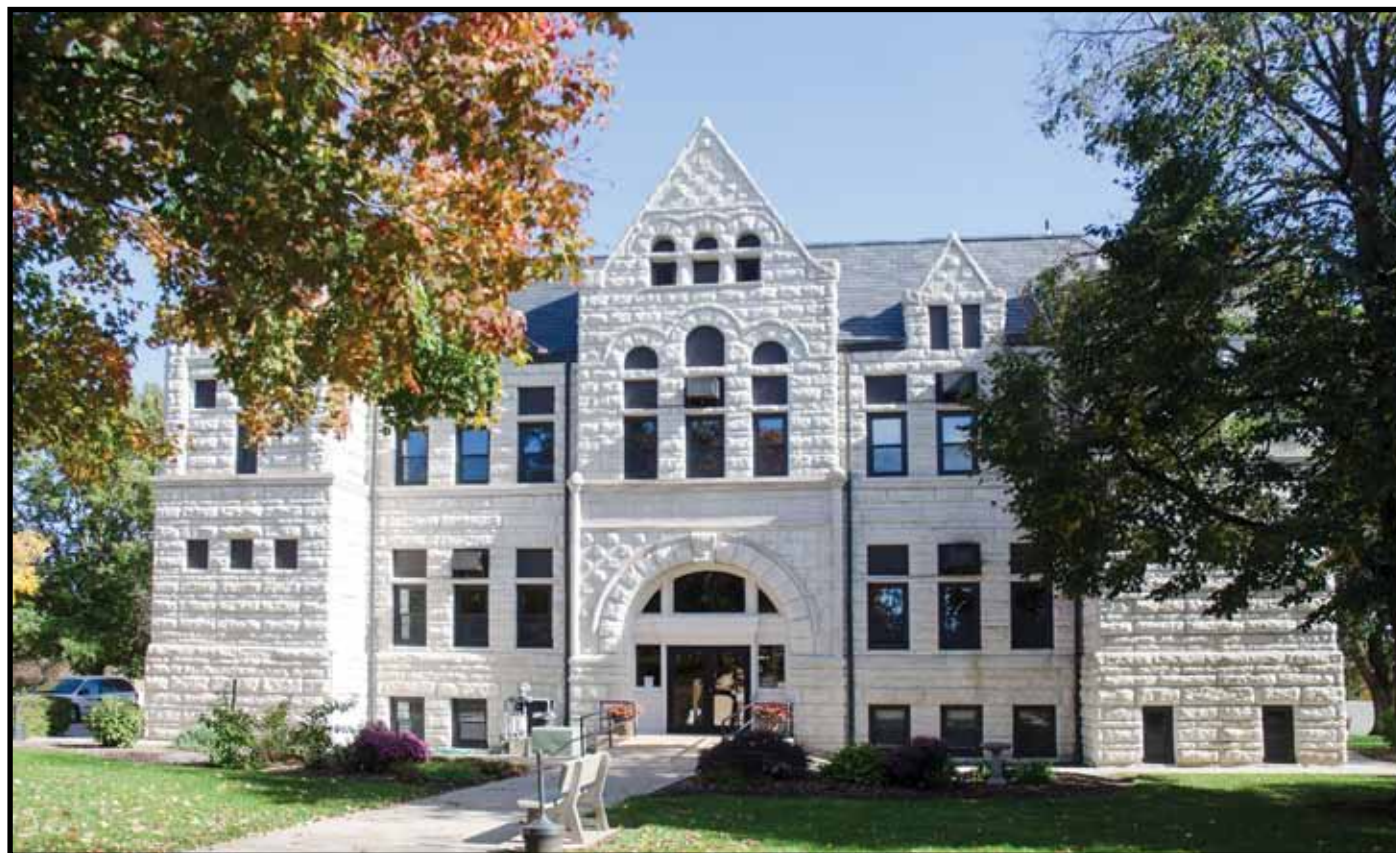
Nemaha County Courthouse, November, 2016
