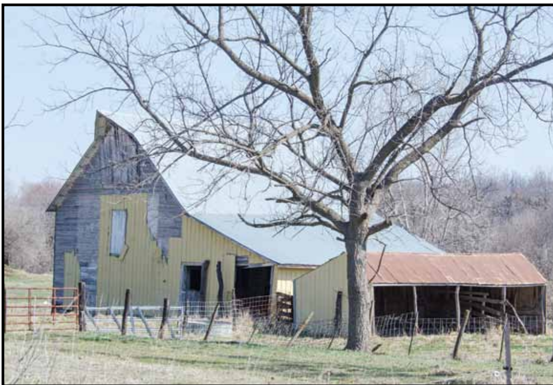
Old Barn in Nemaha County near Howe, Nebraska
